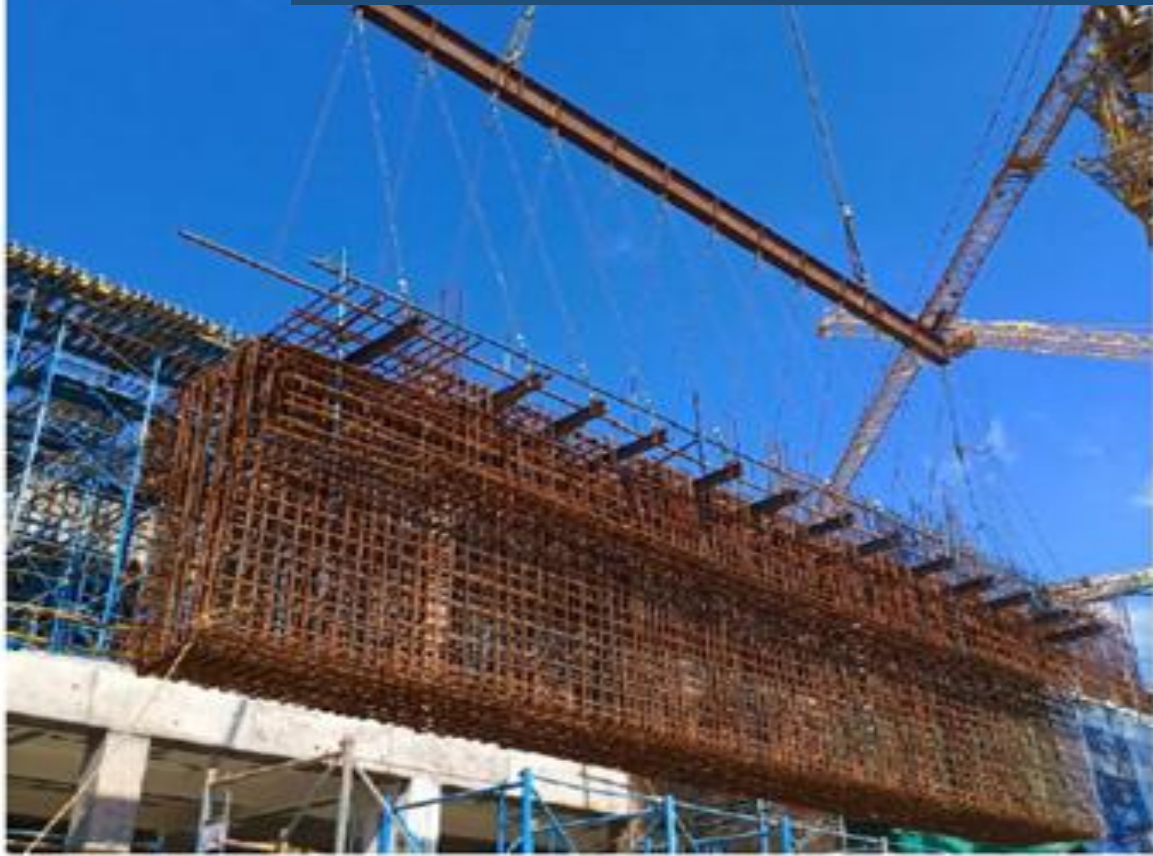
Rebar Cage TB Deck Beam: KKNPP 3&4
